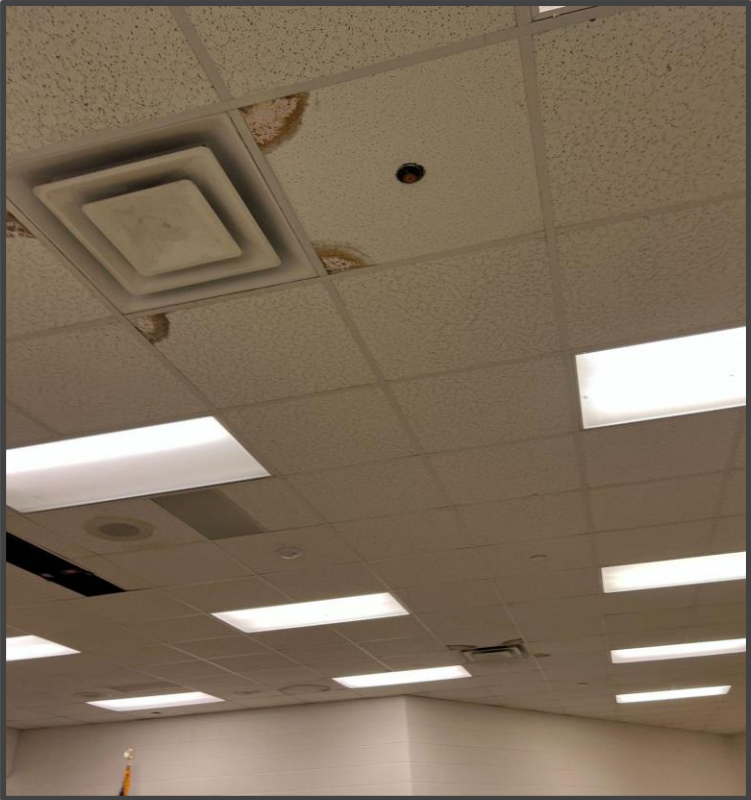
Library ceiling tiles
